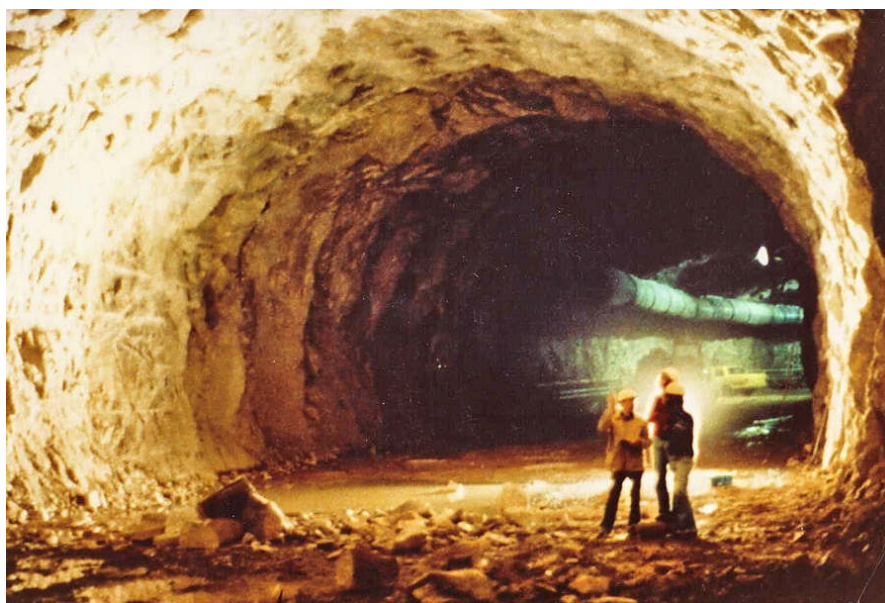
Figure 6 Typical Drill & Blast Tunnel
